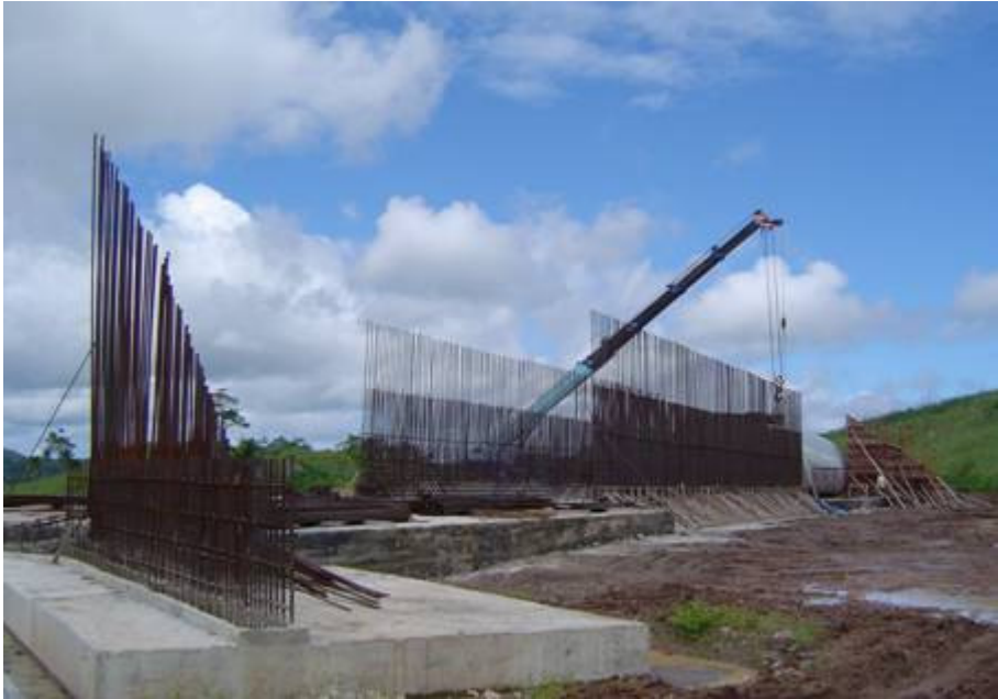
Figure 5: Construction of 6,000t capacity live stockpile with tunnel and retaining walls
