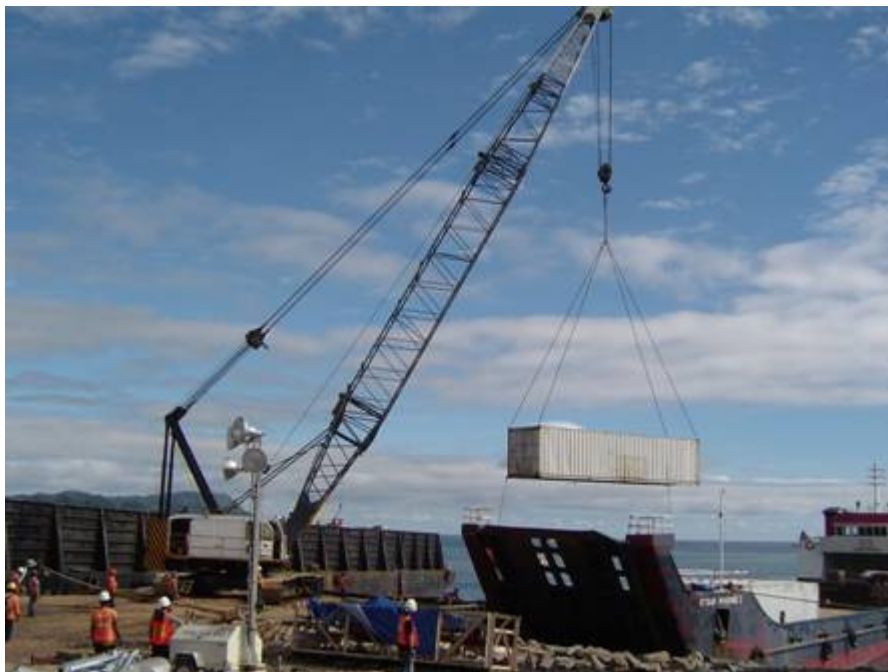
Figure 1: Unloading of one of the final containers of processing plant components
