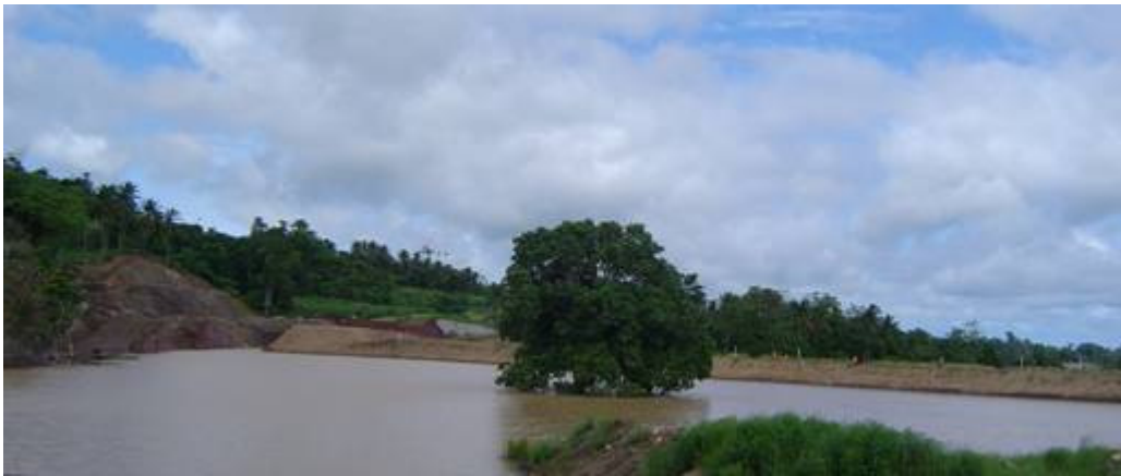
Figure 6: Sediment pond with diversion channel in far distance
