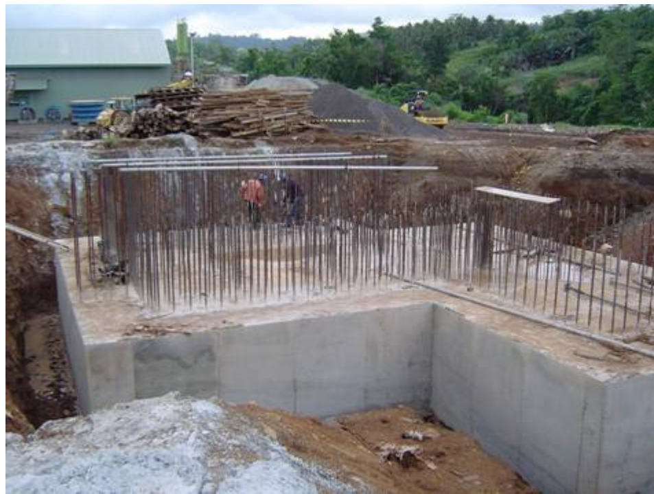
Figure 2: SAG mill foundations
