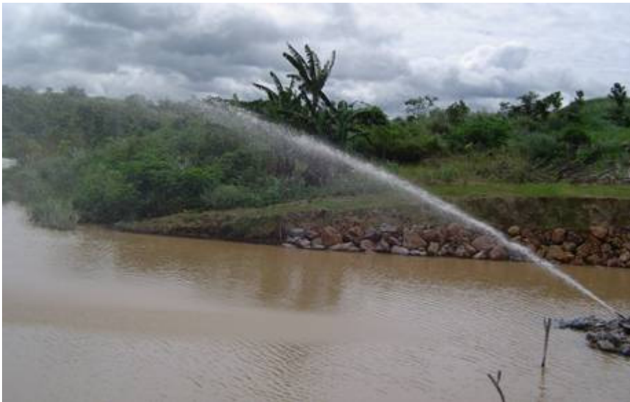
Figure 7: Water treatment dosage point at one of the spillways
